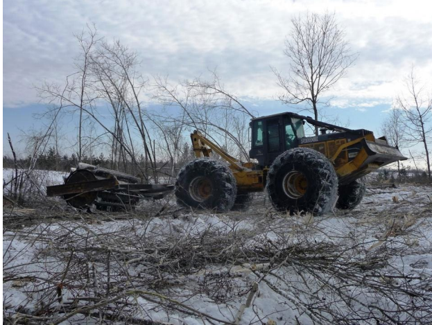
Single Drum Roller Chopper Used for Site Preparation with Frozen Ground.
